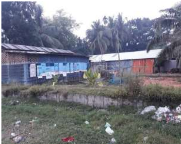
sewage pumping station-5, kasimnagar, Sonadanga
