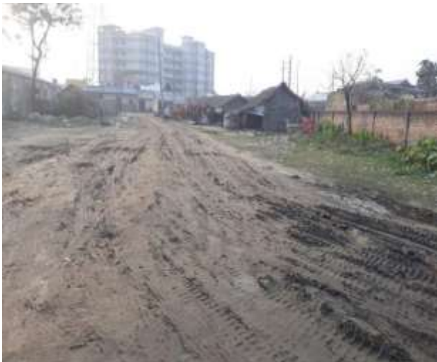
sewage pumping station-3, Lobanchora sluice gate
